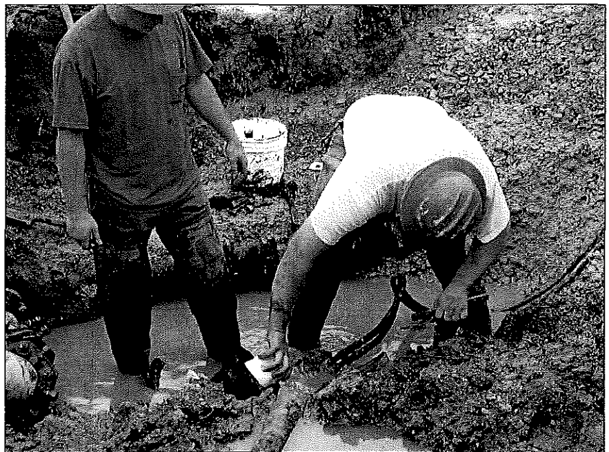
A Fort Scott, Kan. city crew inserts a soft pig into a 4-inch ductile iron line.
