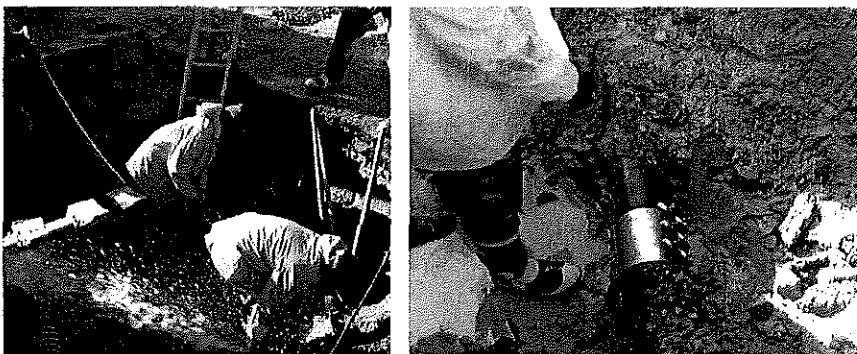
City of Flint Water Service Center employees work to contain and repair one of many main breaks that continues to occur as a part of an antiquated infrastructure system.
