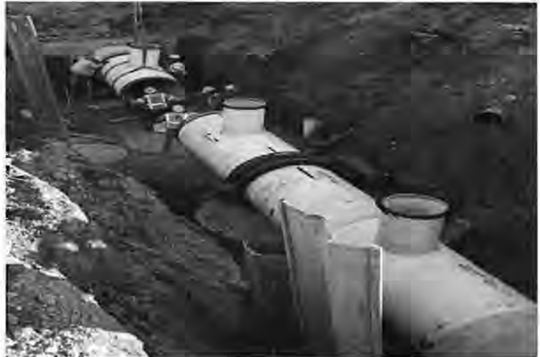
KWA pipeline construction
